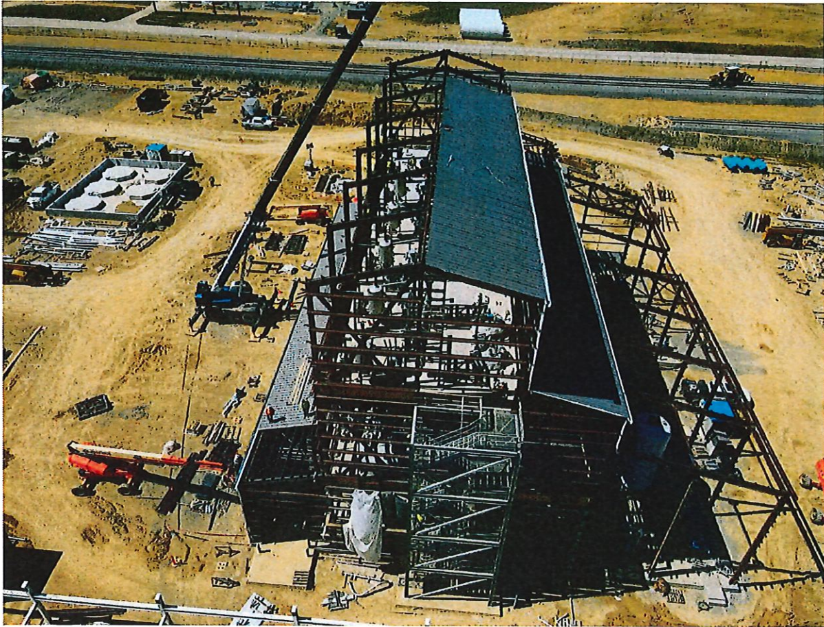
Photo 3: Overhead view of NBR facility
